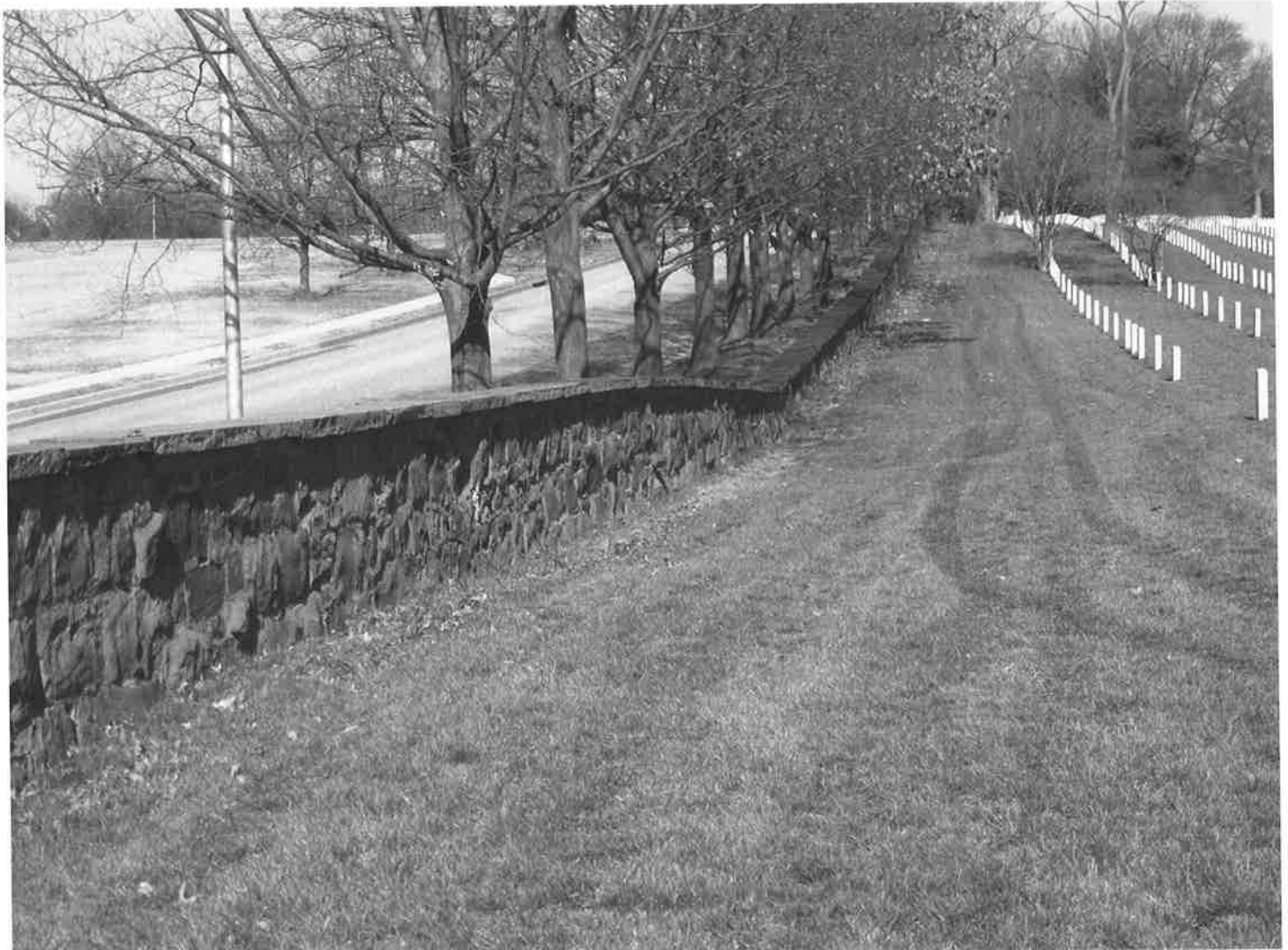
Photo 20. View north along Seneca sandstone boundary wall.
