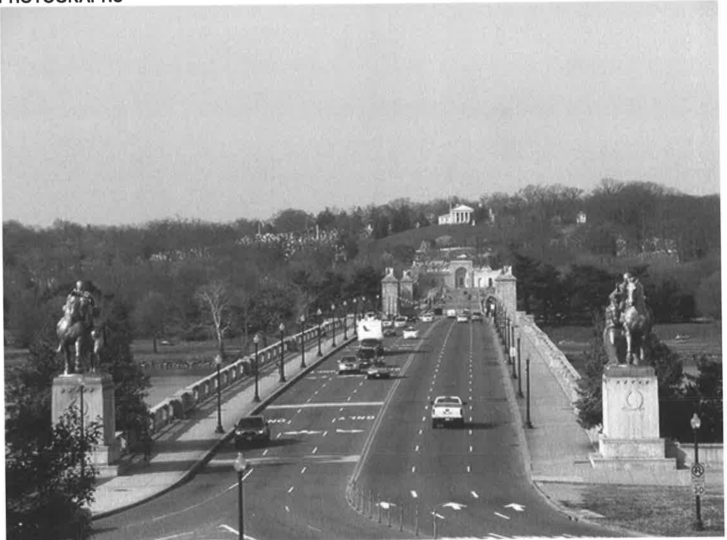
Photo 1. View to the southwest, approach to ANC from Arlington Memorial Bridge.
